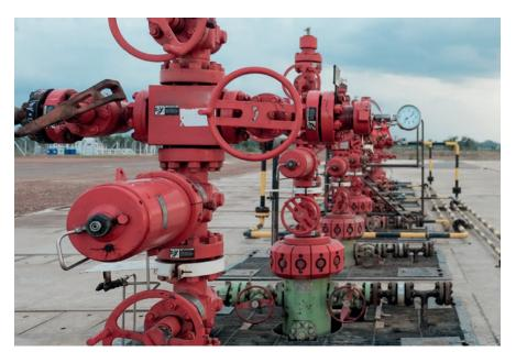
As a part of safety measures, the wellheads are equipped with advanced Safety Gas Sensors to detect harmful gases such as H2S (hydrogen sulfide) and Combustible Gas Detector. These sensors continuously monitor the air quality and trigger appropriate actions if gas concentrations reach hazardous levels, ensuring a safe working environment.
