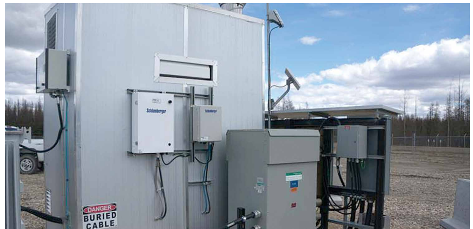
The SCB3 site communication box is assembled with a satellite modem, a CPU control board with memory buffer, a power supply with backup, and field interface connectors inside a small-footprint weatherproof enclosure.
