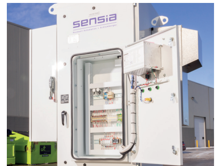
Dedicated Low-Voltages Control Cabinet
