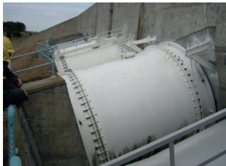
25 foot diameter penstock with transducer feed through with optional weld-o-let reinforcement
