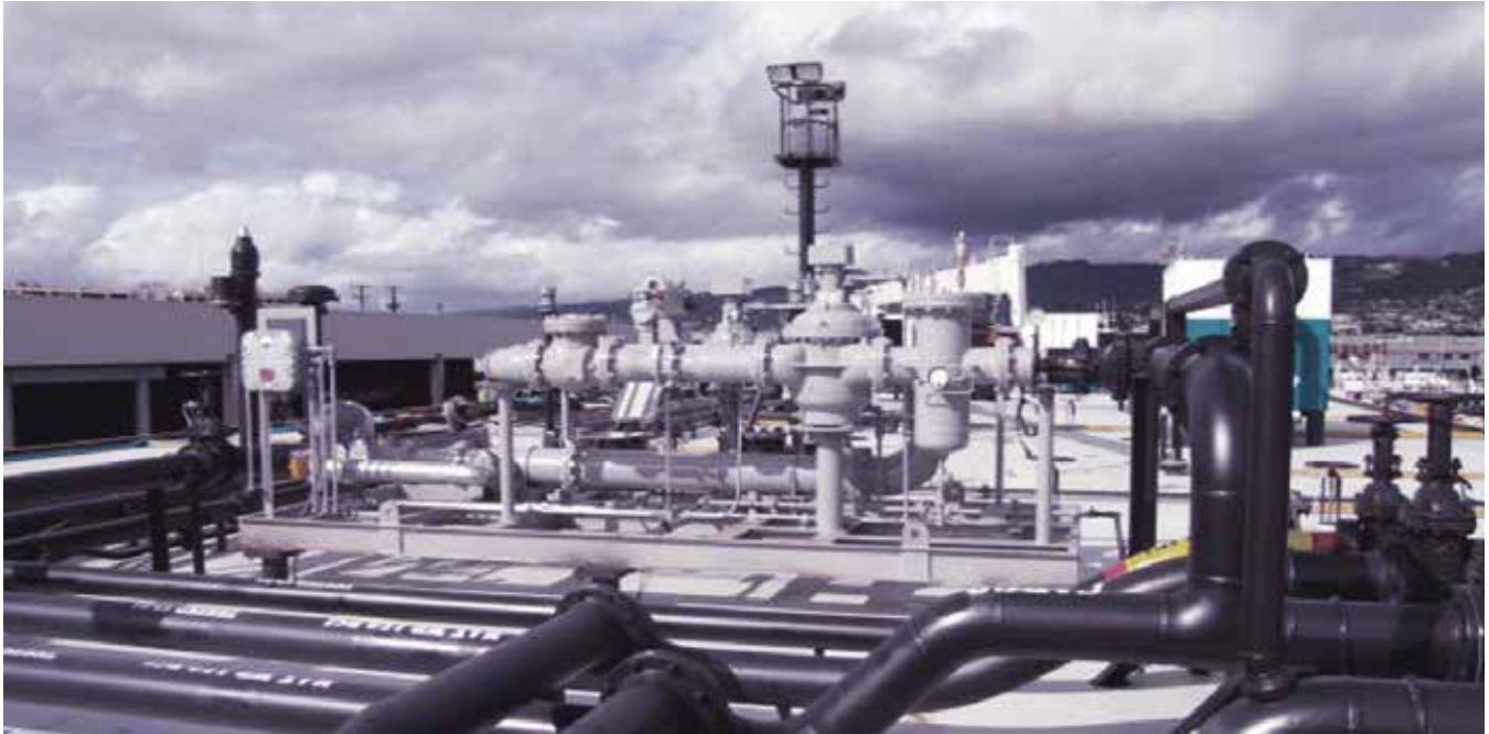
JISKOOT in-line blending system for fuel oil
