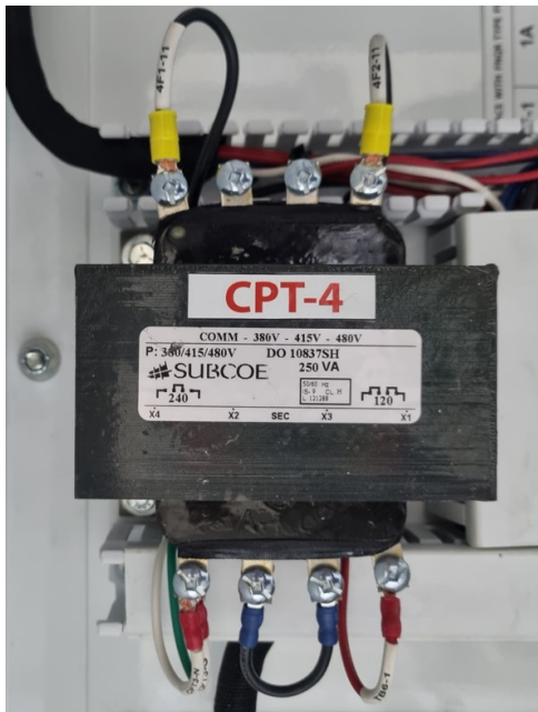
Figure 5-14: 250VA CPT, 380/415/480V primary
