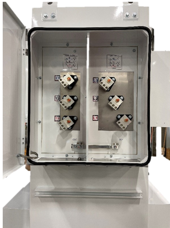
Figure 7-1: Terminals in Power Junction Box
