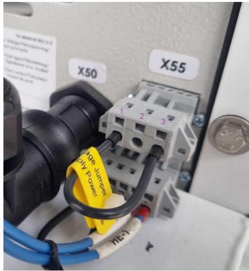
Figure 5-21 – Heat Exchanger Voltage Selection Jumper
