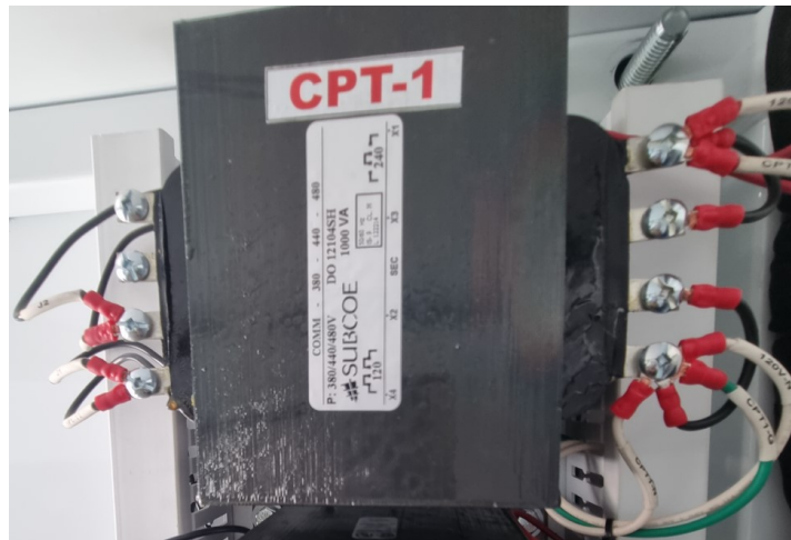
Figure 5-15: 1000VA CPT, 380/440/480V primary
