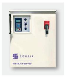
The 10 series have embedded I/O along with three option slots for safety, feedback, communications, 24V power or additional I/O. This flexibility makes the 10 series drive a flexible, cost-effective solution.
