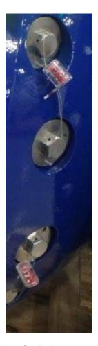
Figure 8.5—Seal wire on meter body
