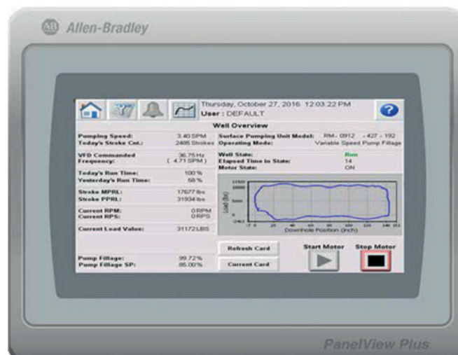
INSTRUCT SRP Intelligent Controller's touchscreen HMI
