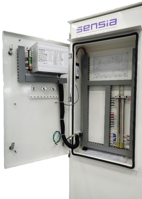
Figure 1.2: INSTRUCT ESP Switchboard Low Voltage Compartment
